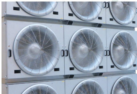
DATA CENTRE (DENMARK)
