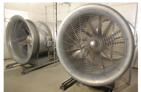
SIMA POWER STATION (EIDFIJORD, NORWAY)
