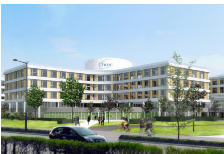
CHIREC HOSPITAL (AUDERGHEM, BELGIUM)
