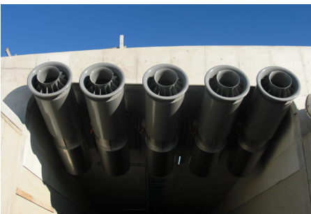
KING WILLEM ALEXANDER TUNNEL (THE NETHERLANDS)
