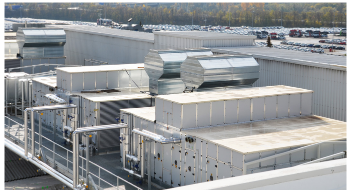
Roof-installed AHUs with ZerAx ® axial fan
